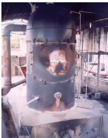
Fig. 5: The boiler foundation and the boiler at Sewagama Rice Mill [2]
