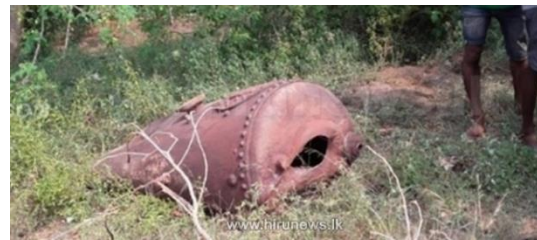
Fig. 8: Exploded boiler at the Valvettithurai poultry farm [12]
