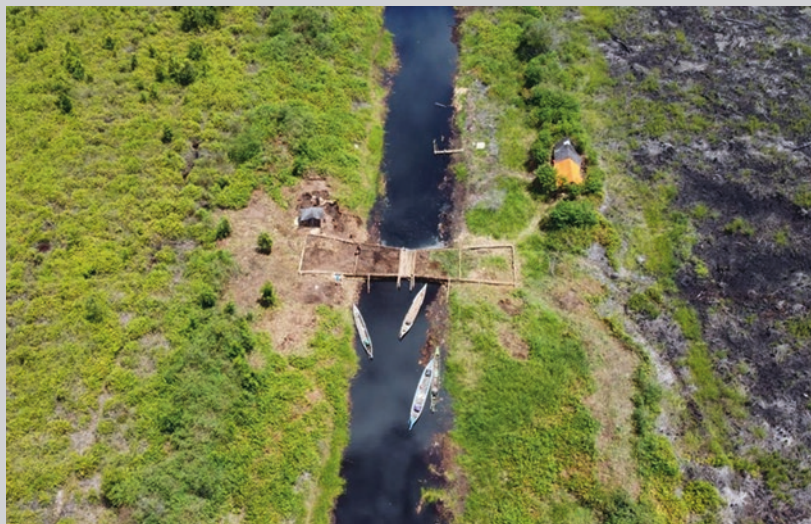
Fig. 7.5 Aerial view of one of the ex-Mega Rice Project Canals, in Central Kalimantan, Indonesia, being blocked by BOSF, to recover hydrology in the area, reducing fire risk and enhancing natural regeneration. (Photo Laura Graham)
