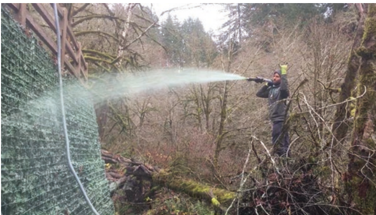
Fig. 9.23 “Hydromoss” application to mechanically stabilized earth wall. (Photo credit Schuyler Hamilton)
