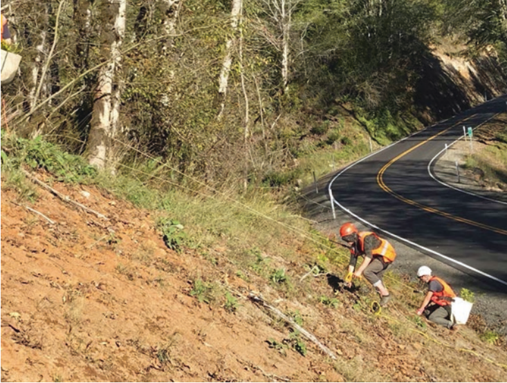
Fig. 9.20 Rappelling to plant on steep slopes on the Nestucca River Byway project. (Photo credit Haley Smith)
