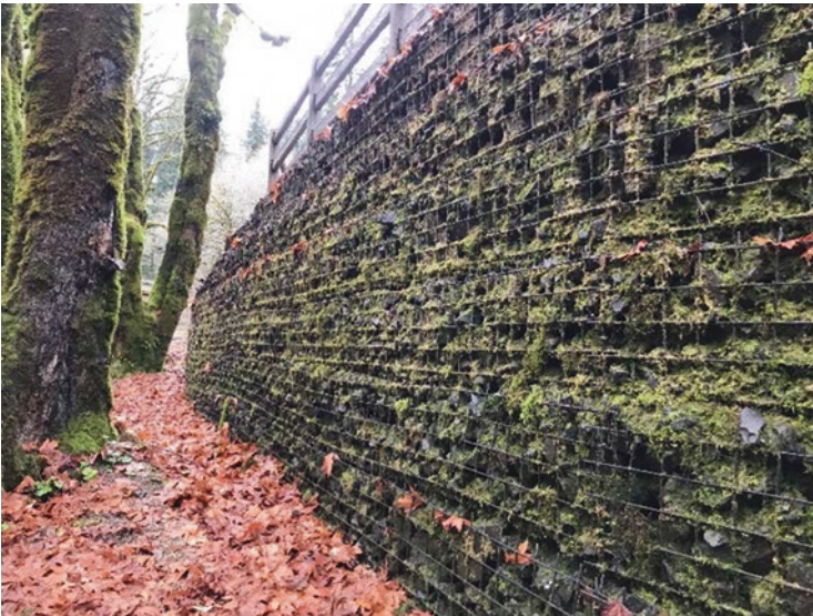
Fig. 9.24 Mechanically stabilized earth wall 1 year following hydromossing. (Photo credit Lee Riley)
