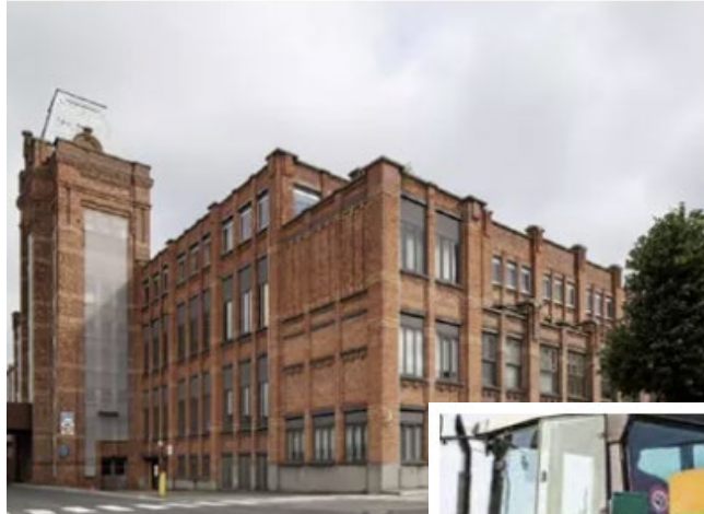
GHENT (BELGIUM) - FLUX MEASUREMENTS FOR BROWNFIELD REDEVELOPMENT Ghent, Belgium: 2020
